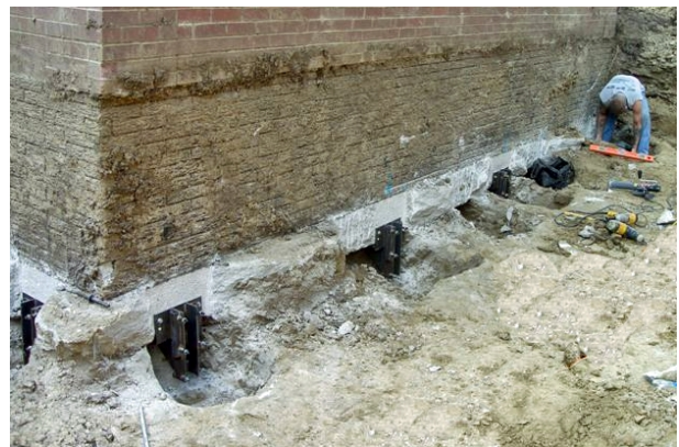
The footings are notched and adjusted to allow the ECP Steel Pier™ brackets to support the underside of the footing.
