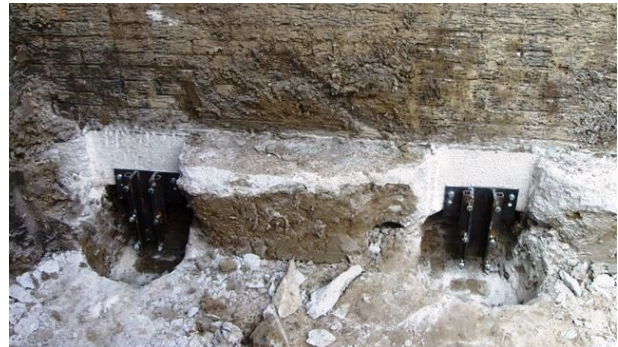
The footings are notched and adjusted to allow the ECP Steel Pier™ brackets to support the underside of the footing.
