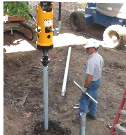
The photographs show a pile being installed with a 12,000 ft-lb motor.
