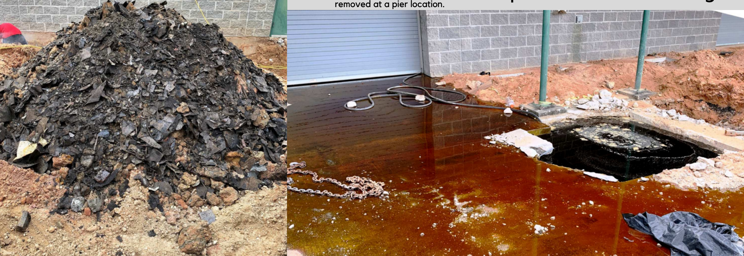
Photos show 2 previously installed push piers, filthy perched water flowing from below the structure and a huge pile of decaying garbage removed at a pier location.
