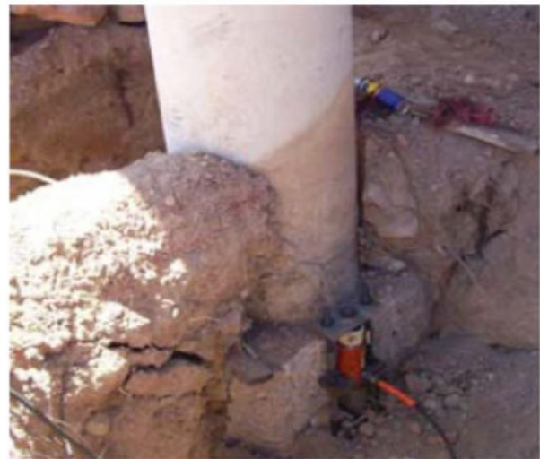
FIGURE 7—INSTALLATION OF TYPICAL ECP STEEL PIERS™ SYSTEM
