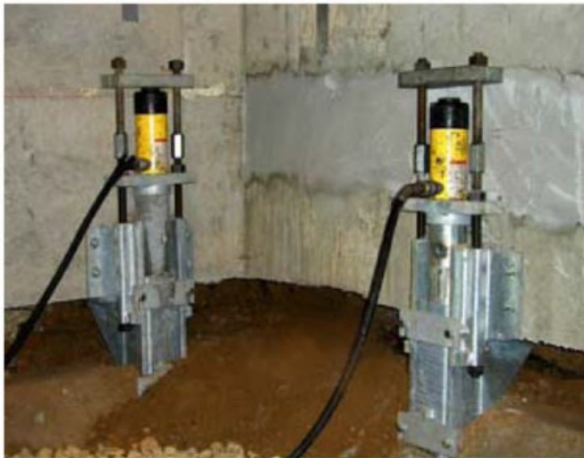
FIGURE 7—INSTALLATION OF TYPICAL ECP STEEL PIERS™ SYSTEM
