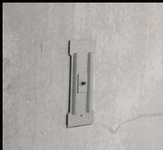
Wall Plate Attached
