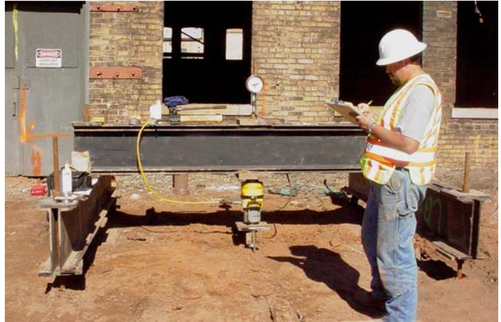
Photo above: A technician records the pile deflections as the test pile is loaded.
