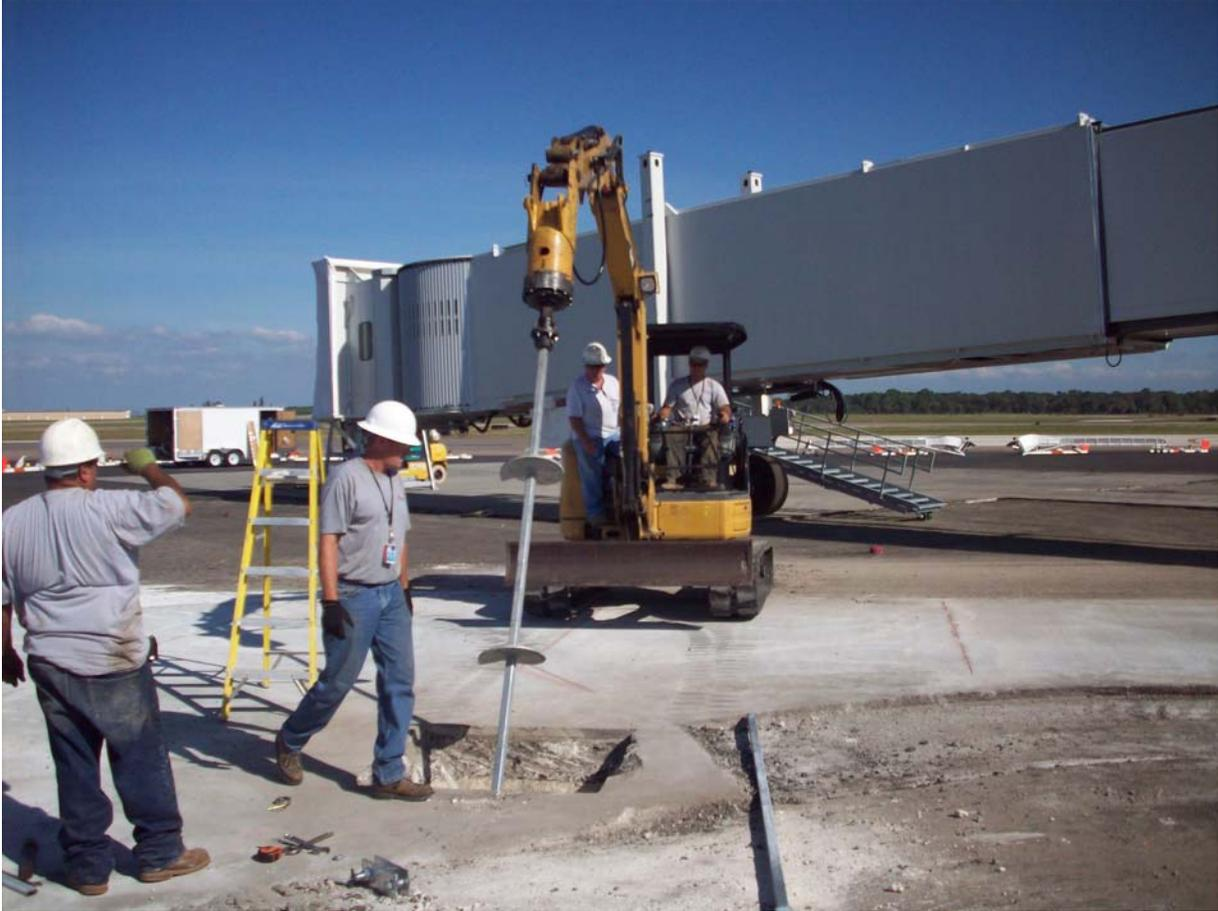
The photograph above and on the previous page shows the installation of the ECP Torque Anchors™ at one of the new passenger bridges. The tieback anchor configuration consisted of three 14 inch helical plates attached to a 1-3/4 inch high strength square shaft. The anchors were advanced into the soil using a 12,000 foot-pound hydraulic gear motor shown mounted to a mini-excavator's dipper arm.
